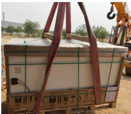
Fig: Packing Box - Adjusting Sling rope for Hoist Handling (Separator – Wooden Plank)
