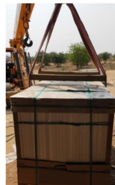
Fig: Packing Box - Adjusting Sling rope for Hoist Handling (Separator – Wooden Plank)
